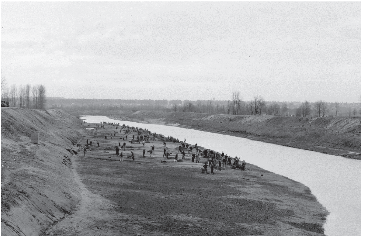
Men working on the Colombia Slough to widen the embankment in January 1935. City of Portland Archive.
